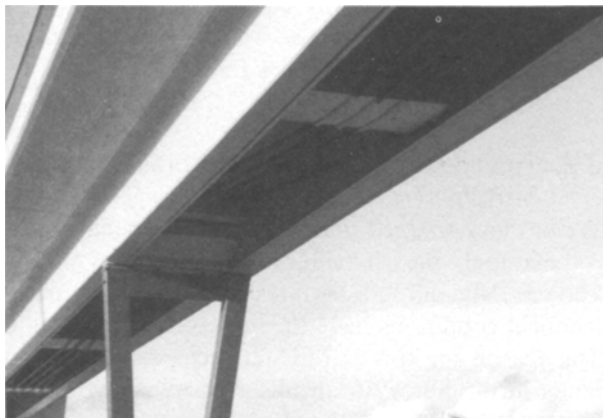
Figure 1 Bottom view of a pedestrian bridge in Berlin Marienfelde.
